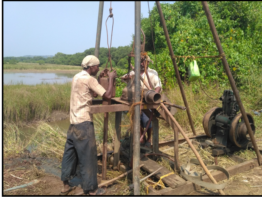
TRIAL BORE IN APPROACH PORTION
