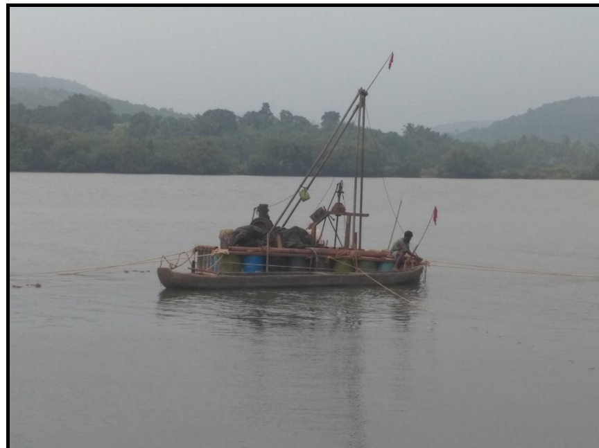
TRIAL BORE IN RIVER PORTION
