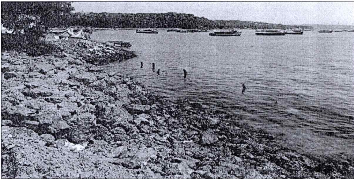
Figure 5-5: Shore protection measures at Coco beach
