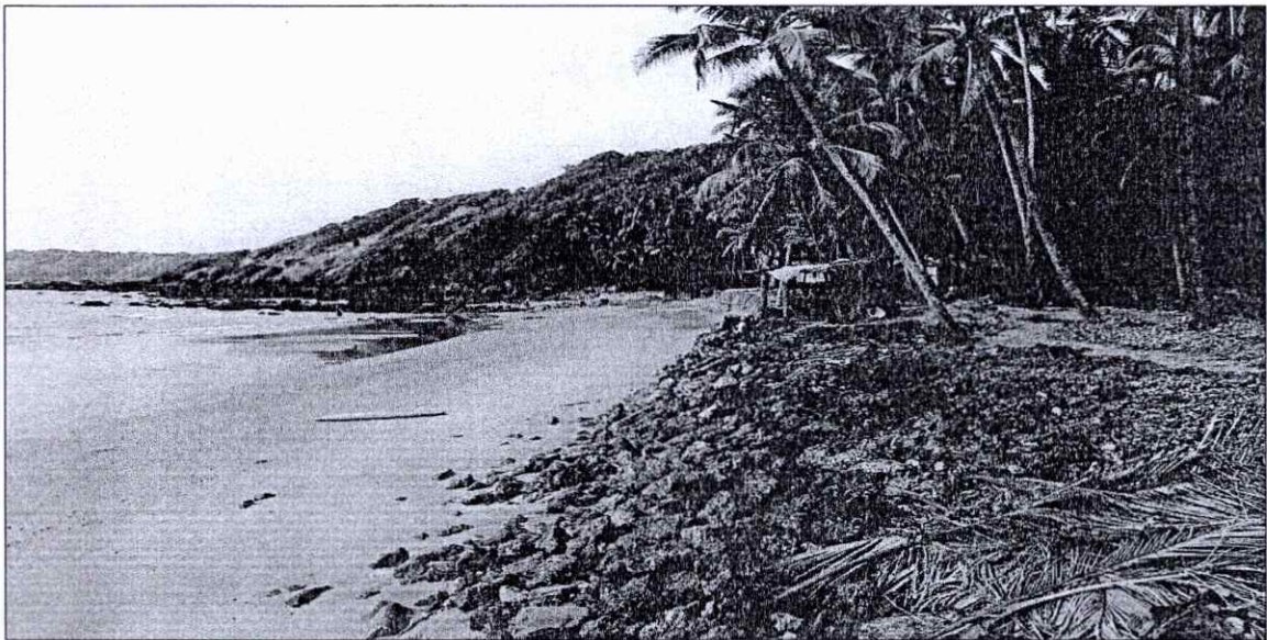
Figure 5-9: Shore protection measures at Canaguinim
