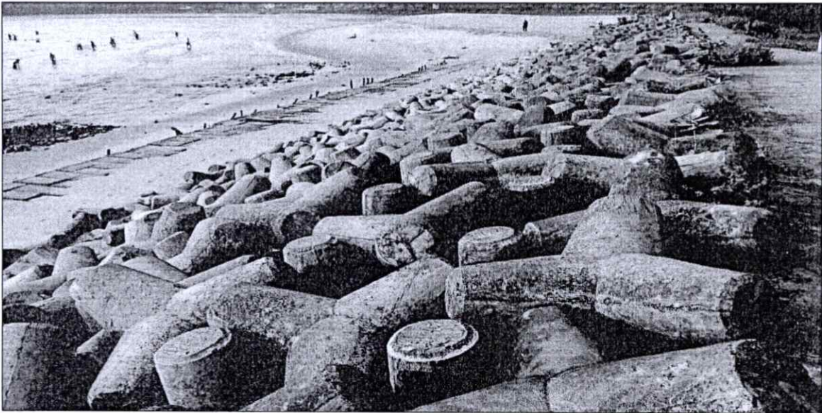
Figure 5-1: Shore protection measures at Keri/Tiracol
