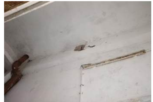
(d) Spalled concrete with R/f exposed along the side of beam of generator room(81)
