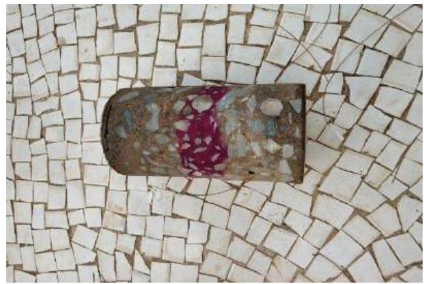
Fig.6.22: Core extracted from ground floor beam (source: group clicked)
