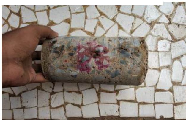
Fig.6.23: Core extracted from first floor beam (source: group clicked image)
