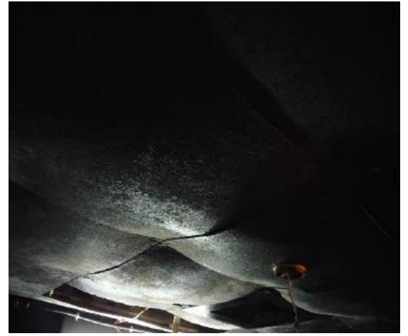
(h) Spalled concrete with exposed R/F in room(9)
