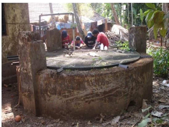
Groundwater monitoring wells
