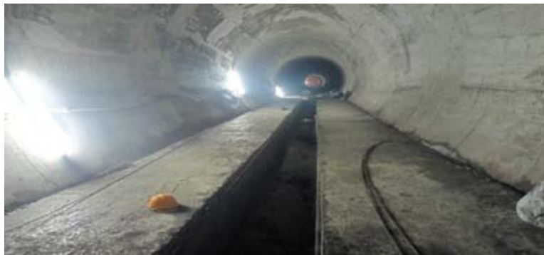
Lining of Escape Tunnel T13 completed
