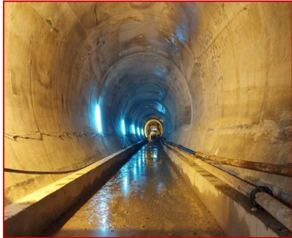
Lining of Escape Tunnel T13 completed
